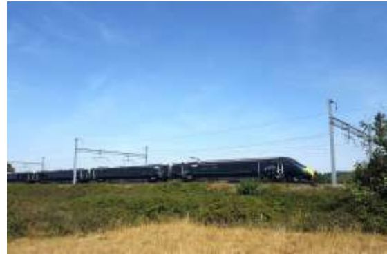
Electrification of railway with new electric train
