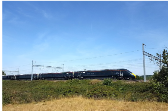
Electrification of railway with new electric train
